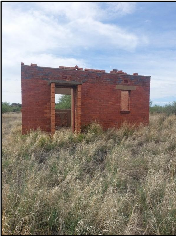
Figure 7.6. View of a partially demolished structure at KG001. There is no roof, windows or doors and only partial walls remain. Additions and alterations to the structure are also visible
